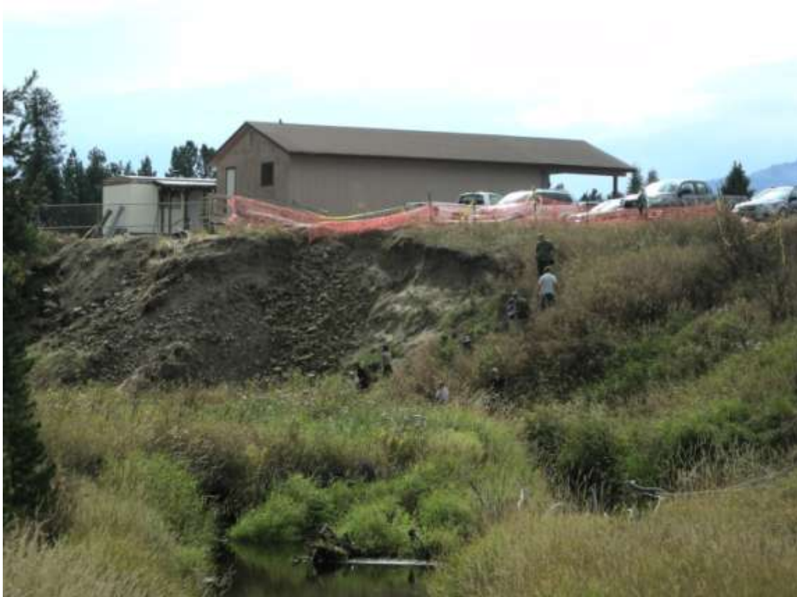
Boulder Creek Eroding Bank- Before Project
