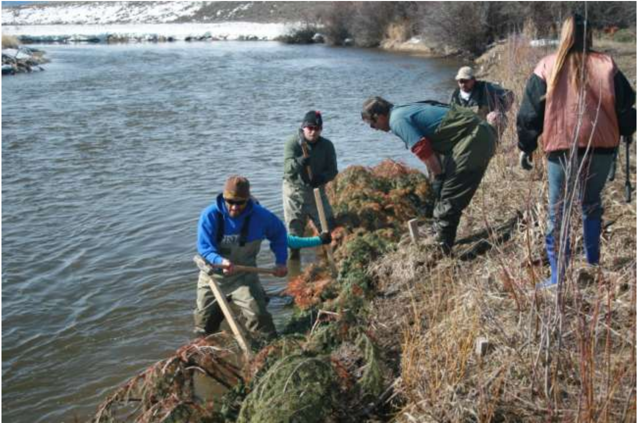
Teton Valley TU and Teton Regional Land Trust personnel use native firs as bank stabilization on Fox Creek
