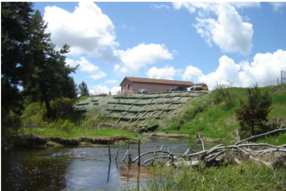
Boulder Creek after Log Grid Installation
