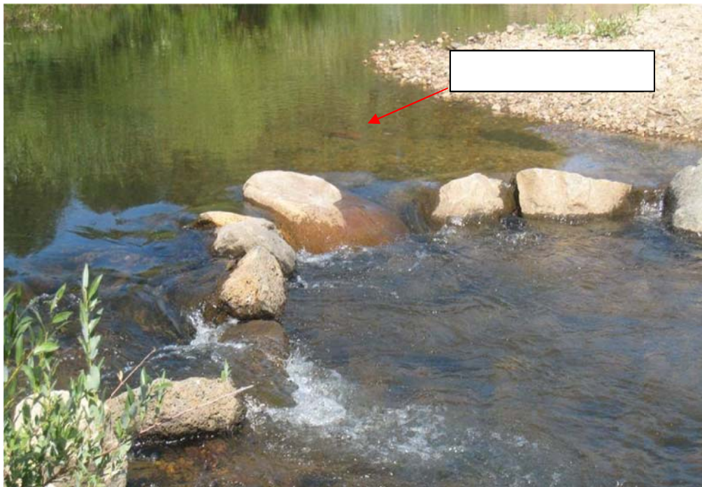
Photograph 6. An upstream facing “V” structure showing a kokanee spawning just upstream from the structure.
