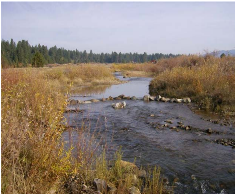
Photograph 4. A typical upstream facing “V” structure right after installation
