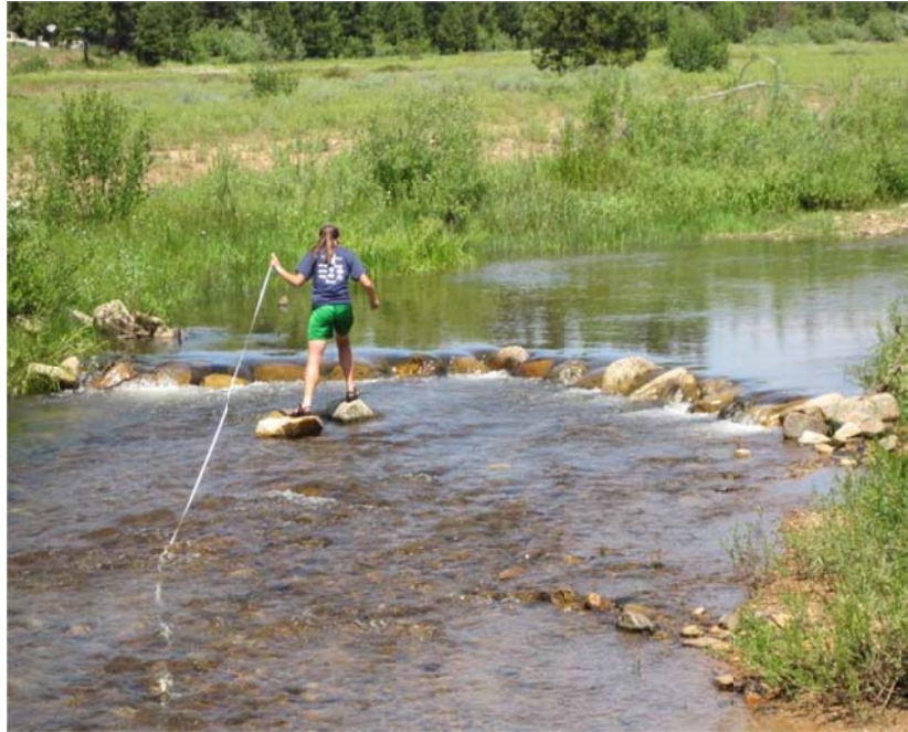
Photograph 5. A upstream facing “V” structure after one year of spring high flows.
