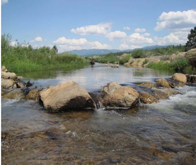
Photograph 3. The same downstream facing “V” in Photograph 2 after one year of spring high flows, showing a long upstream dam pool.
